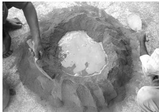
Add water only once a uniform gray color is visible.
