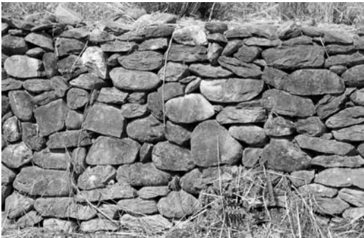
All size bolder stone try masonry wall
