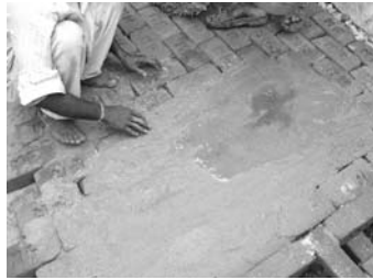
Filling the brick joints with wet sand
