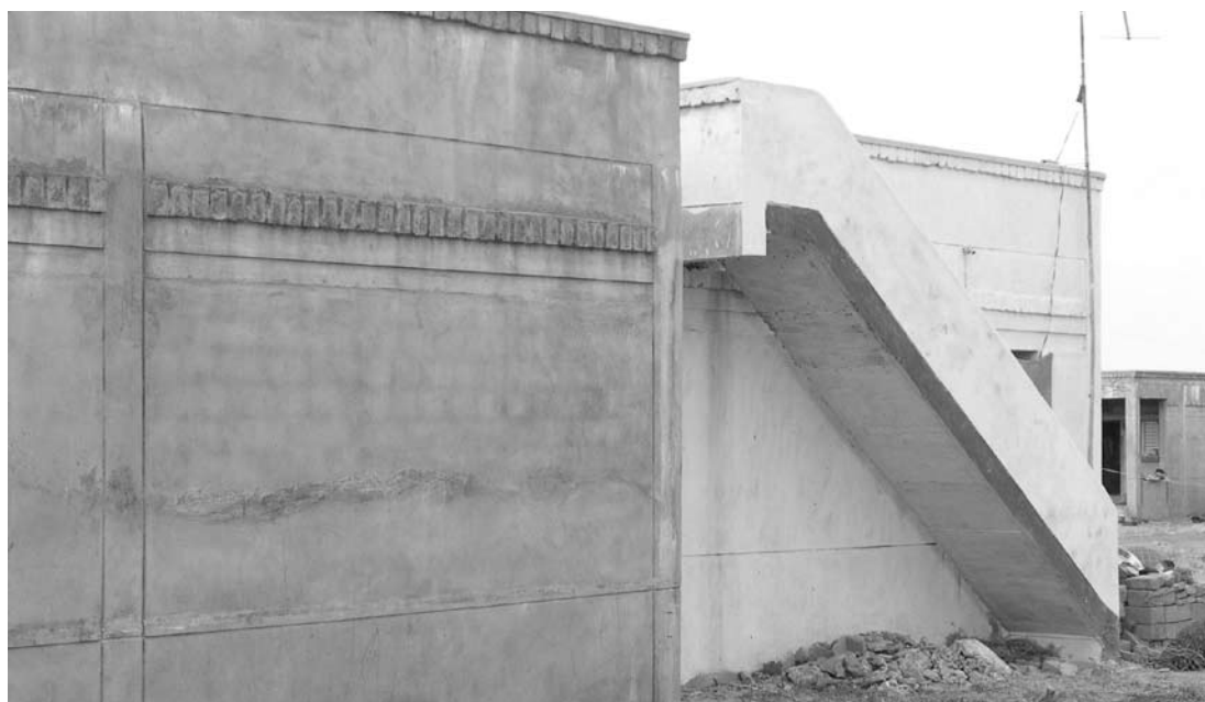
Wall plastering and decorative structure design
