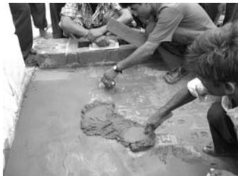
Placing the cement mortar
