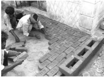
Laying bricks into a bed of sand
