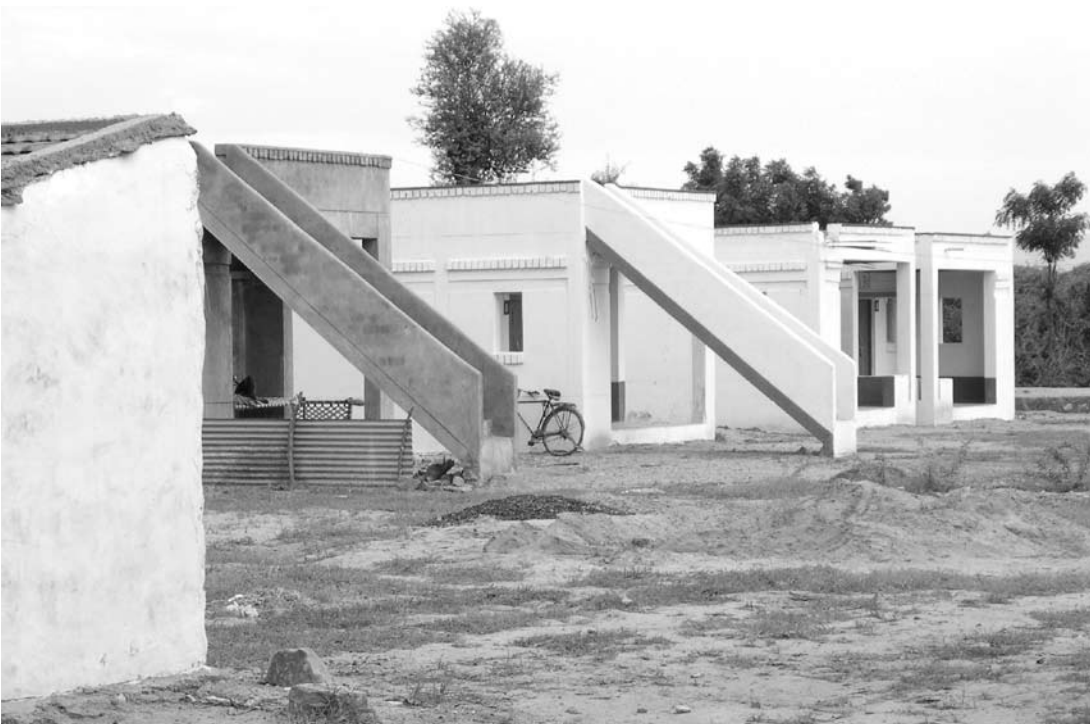
External stair construction, provides safe access to roof area
