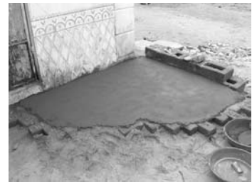
Brick bat floor example completed
