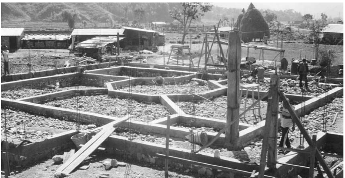
Completed plinth beam of a building
