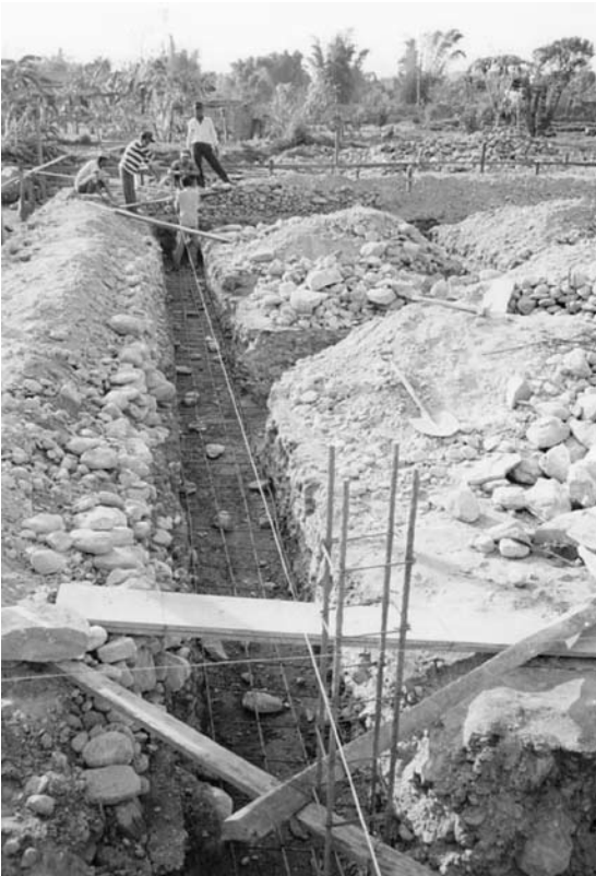
Steel reinforcement placing in foundation excavation
