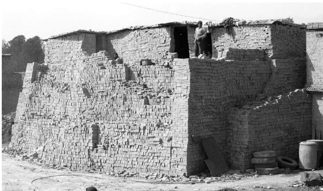
Piling up of common bricks at production site, ready for selling
