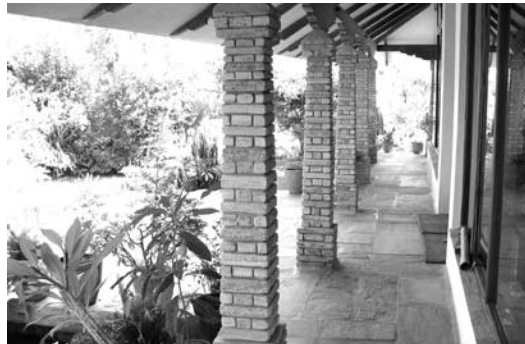
Sized stone pillar construction
