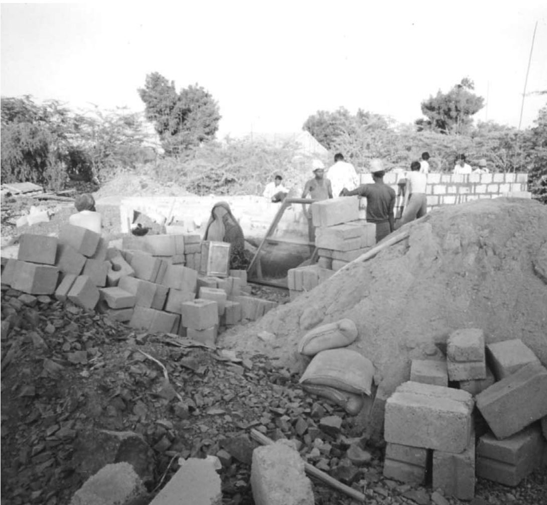
Building material compilation at site (sand, grave, cement, concrete blocks)
