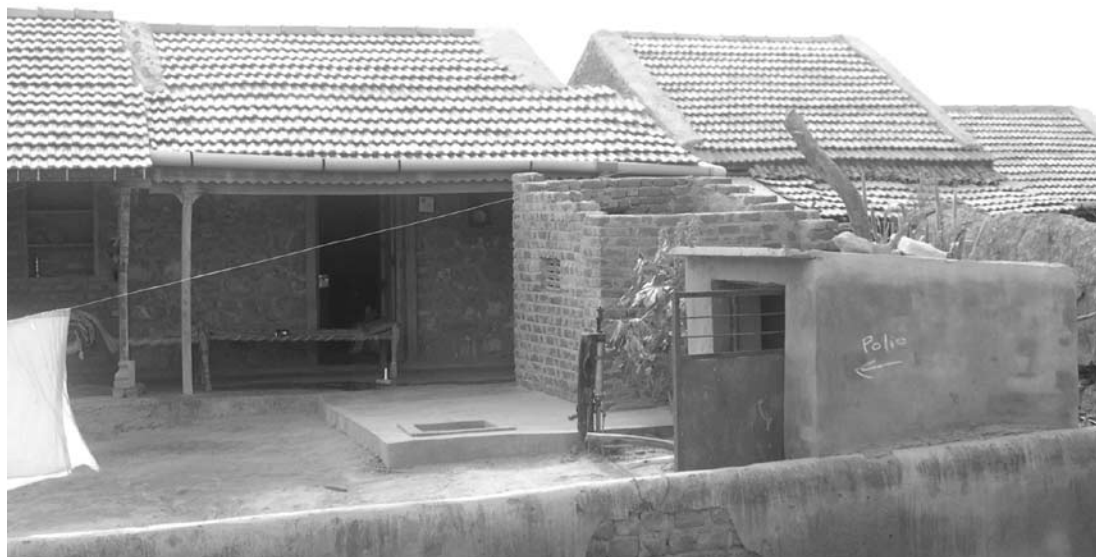
Clay tile covered roofs for rural housing scheme
