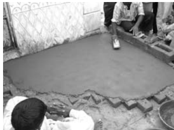
Prepare the floor top finish
