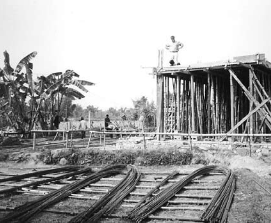
Steel bars properly stored at construction site.
