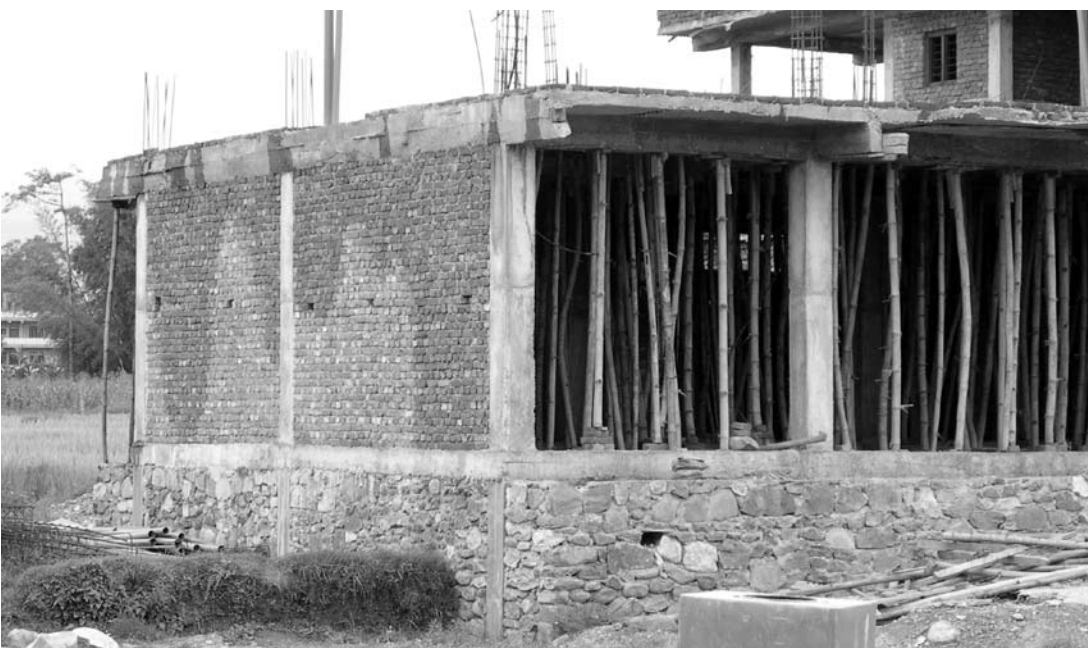
Plinth construction height up to ground floor level
