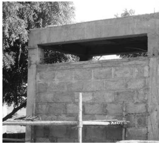
CHB wall construction used in earthquake resistant house design
