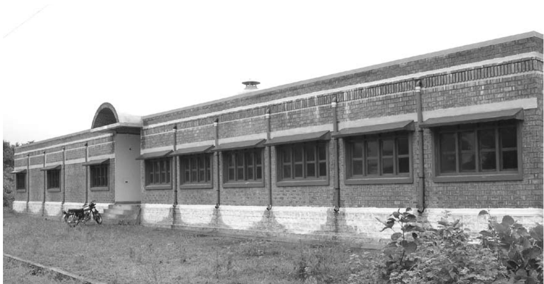
Building with many windows providing desired ventilation and light
