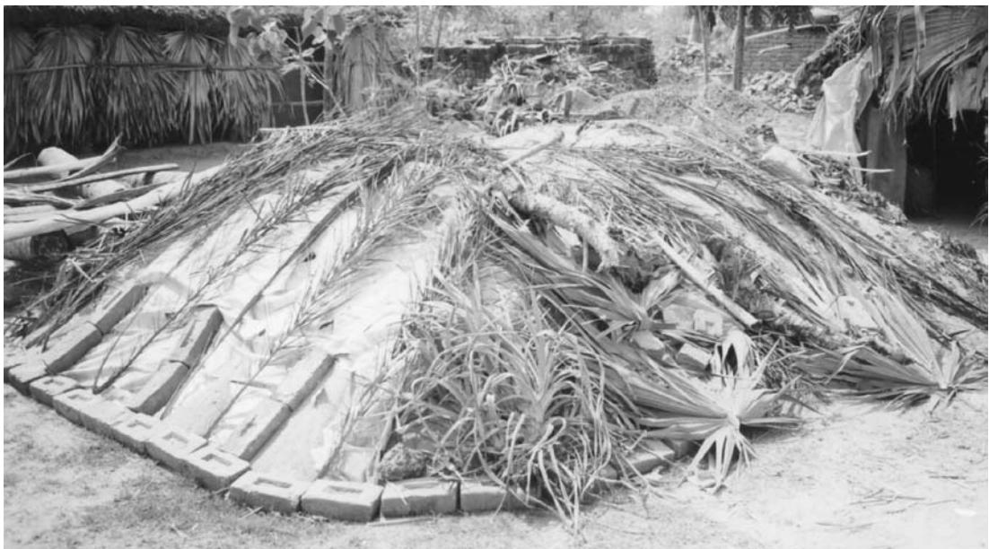
Sand deposit properly covered and protected from being contaminated
