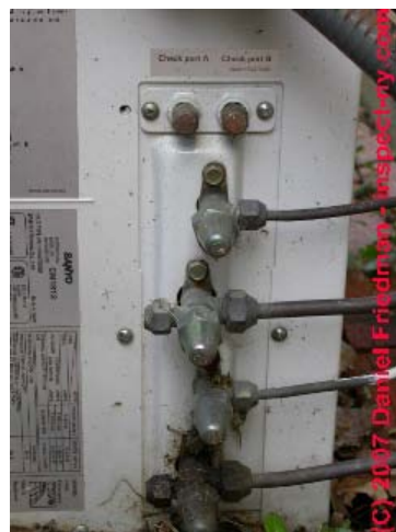
HVAC servicing and repair.
